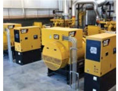
*Located behind the new 17,000 square-foot office of Lehi City Power, the Broadbent Generation Facility first opened in March 2018. It has three Cat G3520H generator sets that produce 7.2 MW of power during times of peak demand, when energy prices are high.*
